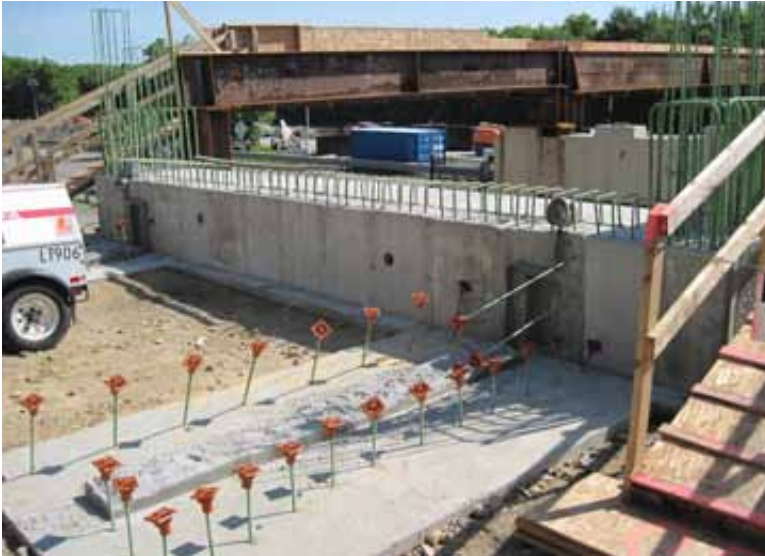
Existing abutments were replaced with two concrete stub-type abutments supported on steel piles.
