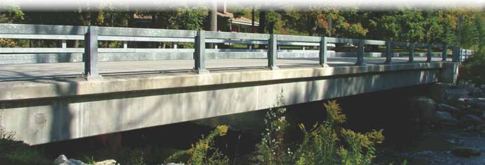
An adjacent precast, prestressed concrete box beam bridge with top-mounted metal traffic railing located in Erie County, N.Y.
