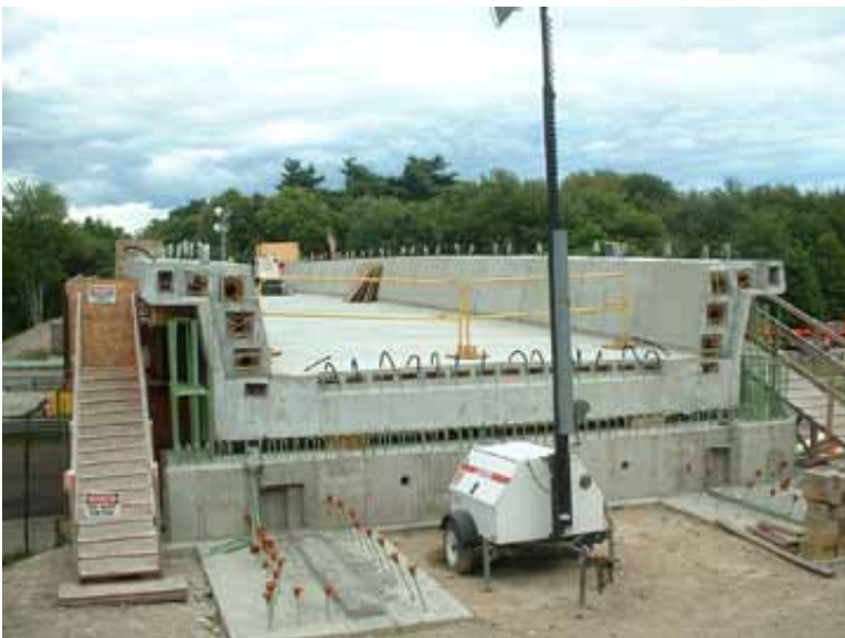
To avoid deflection issues resulting from unequal weight distribution, all of the precast concrete segments were placed onto the temporary erection beams prior to their actual assembly.
