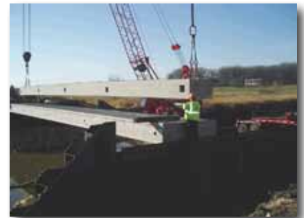
The erection of an adjacent precast, prestressed concrete box beam bridge on steel sheet pile abutments. This is a demonstration bridge in Blue Earth County, Minn.
