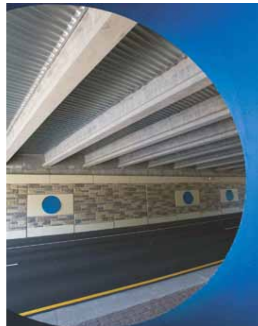
Hand-stained MSE panels and circular cutouts reflect the bridges' intricate, custom design.
