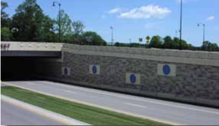
Unique detailing is the hallmark of these bridges. MSE wall panels with ashlar hand-stained finish are punctuated with smooth circle panels where the circles are canted 2 in. in and out from the panel surface. Photos: Henry G. Russell Inc.
