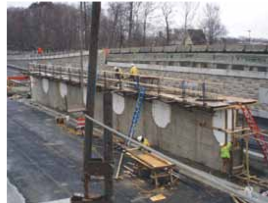
Center piers are cast-in-place concrete frame bents on driven piles.
